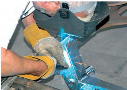
10) After all of the measurements were made and the crossmember was located correctly, it was tack-welded to the frame.
