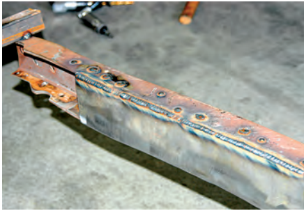
7) Here's what the framerrail looked like after it was boxed. This strengthens the frame at the point where the crossmember will be installed. Without this, the frame could tear from stress over time.
