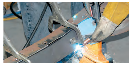
6) O'Bryant decided that it would be better to use a pair of hand clamps to secure the boxing plate before the welding was done. He started by tack-welding the section to the frame at the front and rear.
